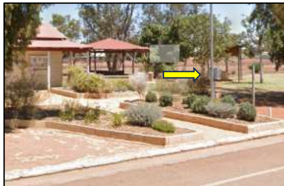
(ref: Google Maps) 3-phase power upgrade conversion to the existing switchboard located between the public toilets and verge on Fowler Street.
