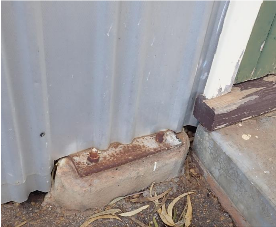
Figure 11: Typical column baseplate and concrete footing.
