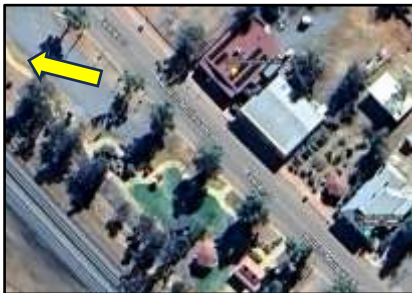
(ref: Google Maps) Proposed Site 2 for EV Charging Station.
