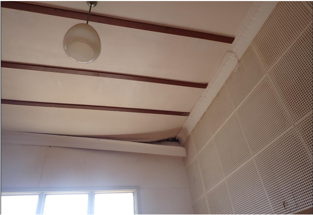
Figure 5: Northeast corner ceiling.
