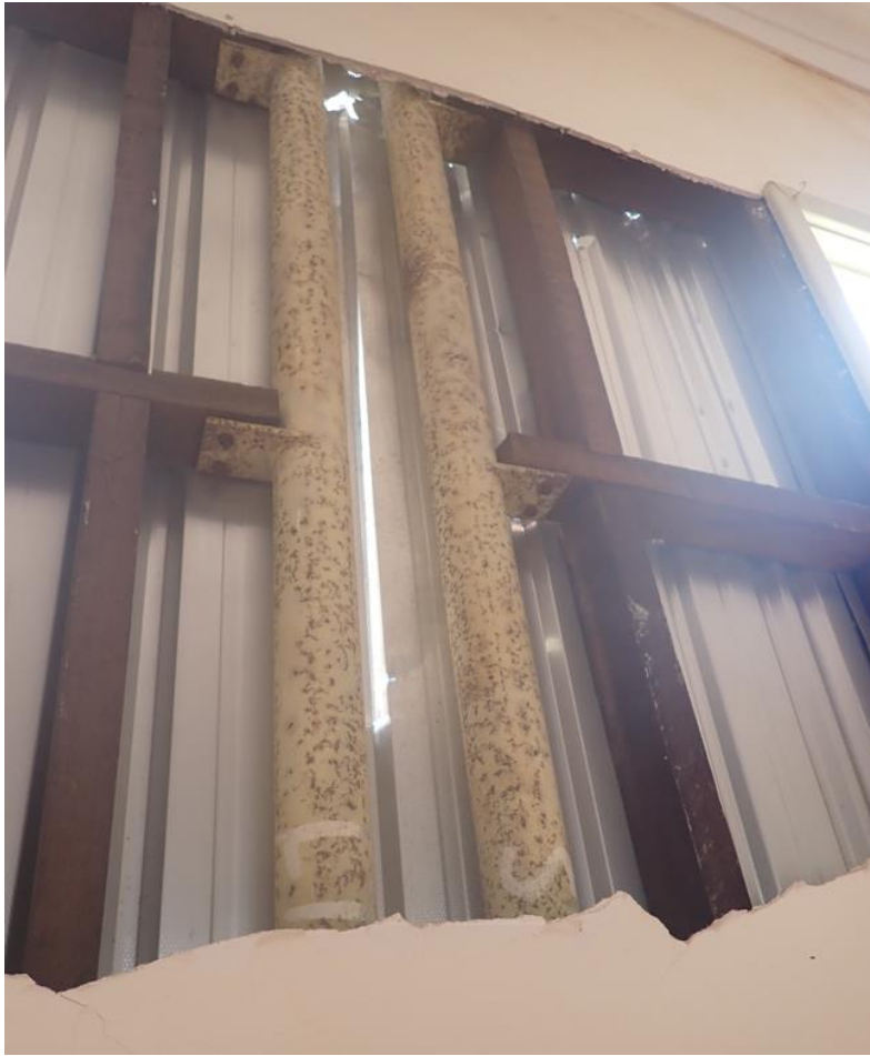
Figure 7: Side by side CHS columns and hardwood timber wall framing.
