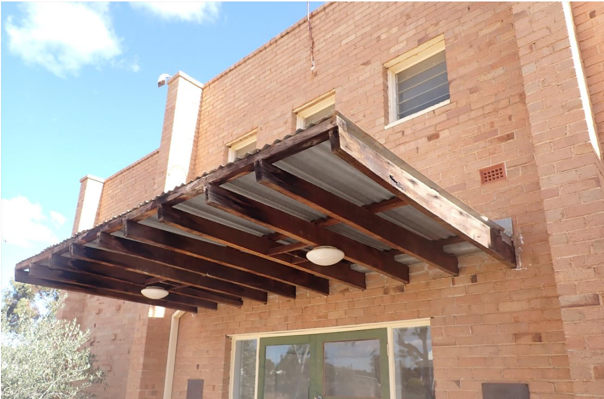
Figure 18: The Cantilever timber entrance roof.
