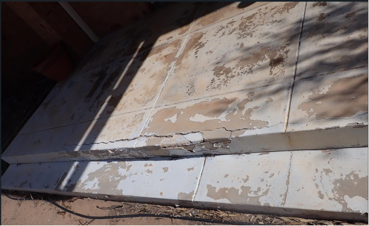
Figure 19: Slab cracking.
