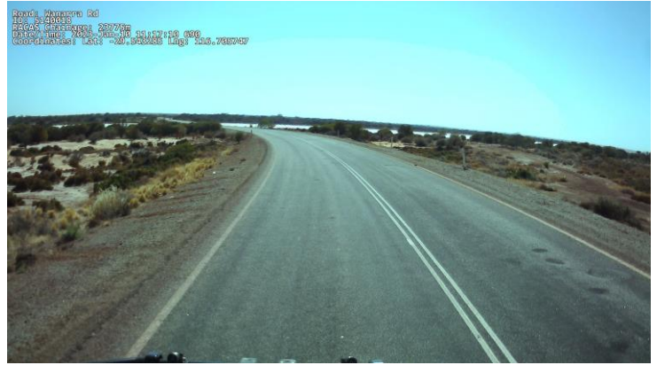
Figure 2: Wanarra Rd potholing
