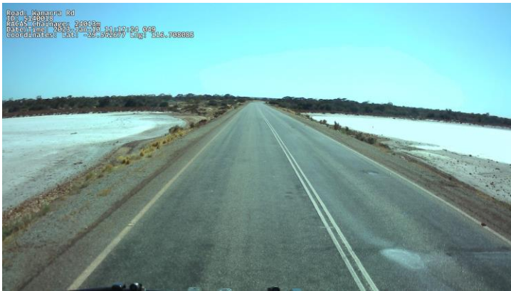
Figure 3: Wanarra Rd potholing
